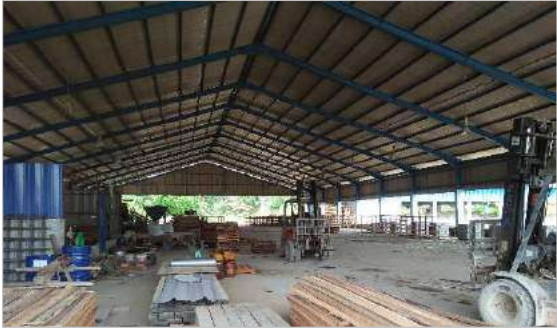
Atan Bina Hardware Sdn Bhd (Cement Products)
